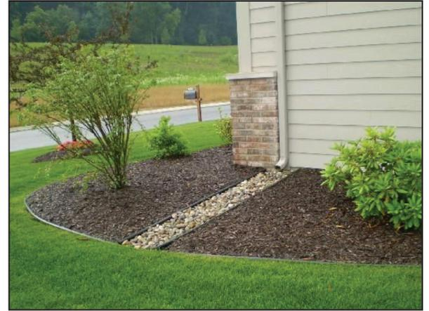
Figure 3. Gutter downspout discharging to lawn.
